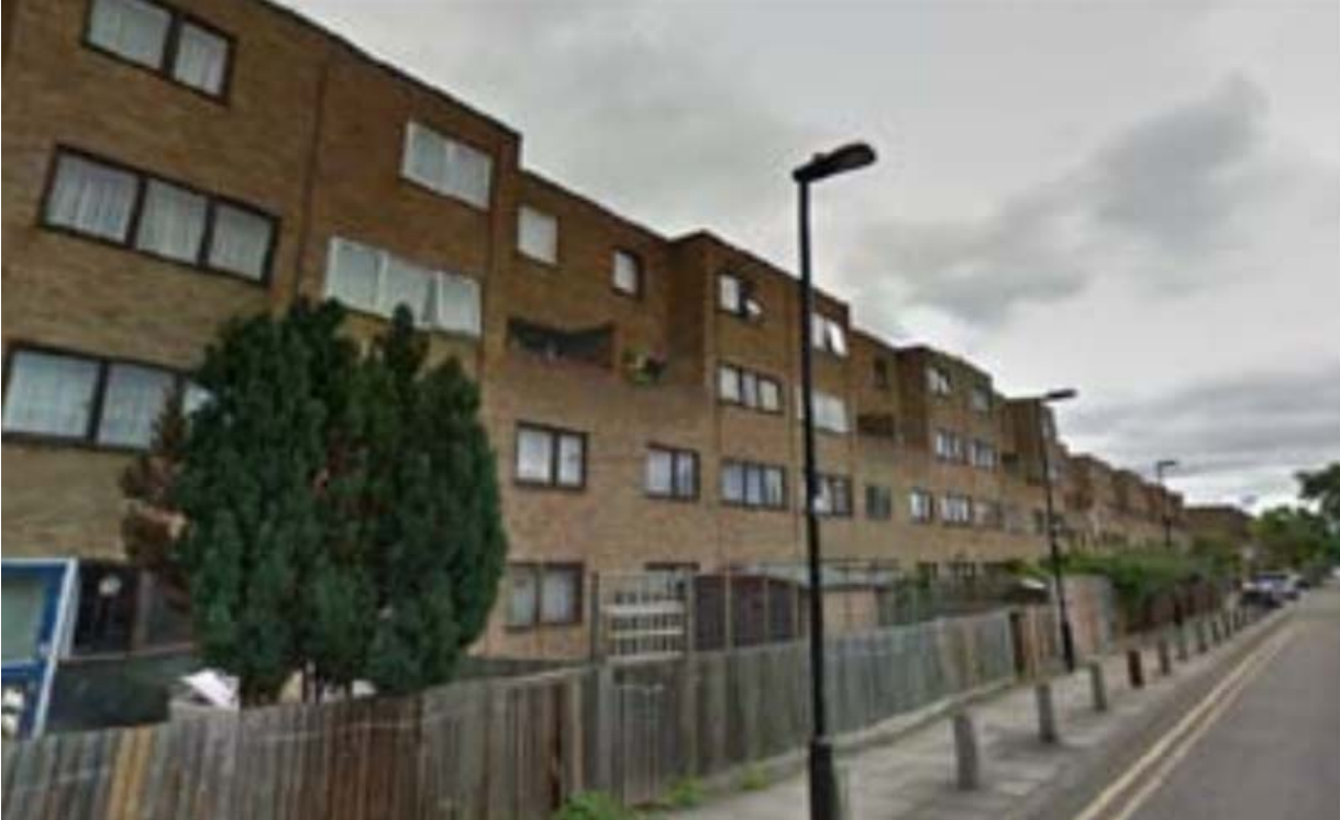
Tamar Way 4 storey residential block to the north of the site
